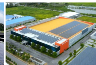
Solar panels at Hanwha Vision Vietnam
